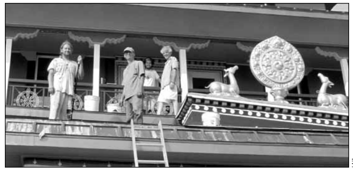
Kirk, Steve, Jeff, and Andy restoring the roof
