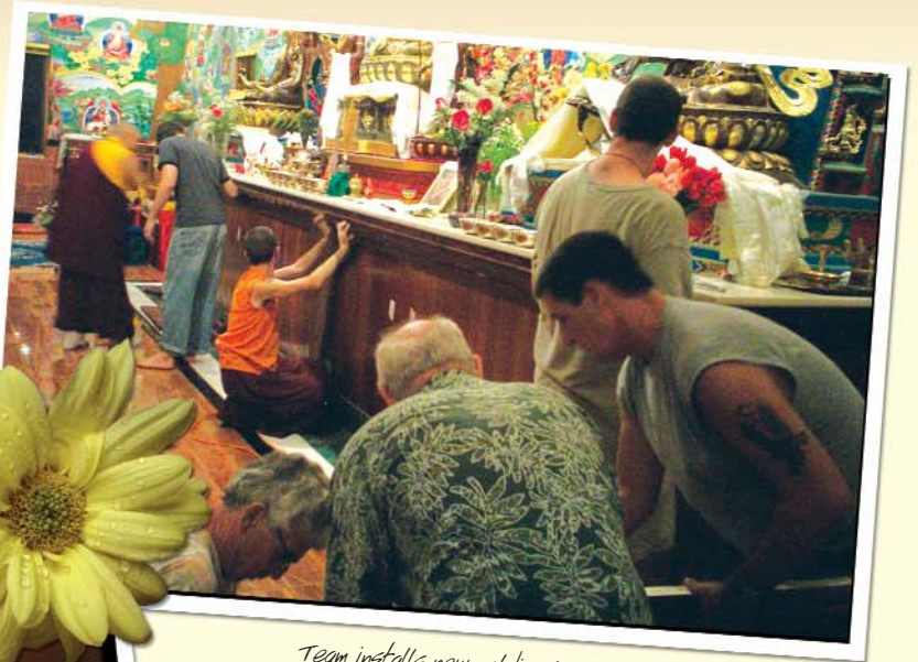
Team installs new molding in main shrine room.
