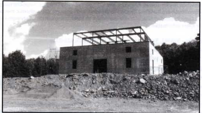
PHOTOS COURTESY OF RON WAGNER
